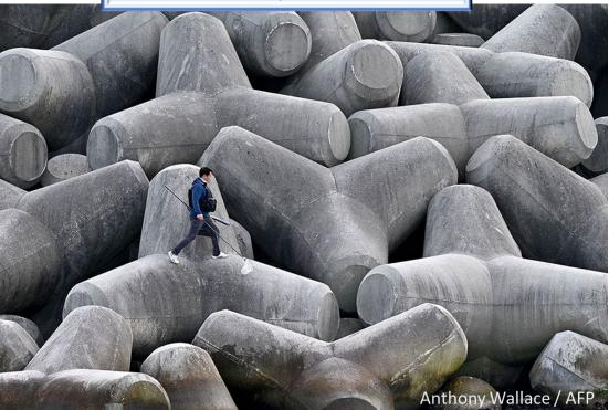
An angler walks on concrete tetrapod wave breakers, whose shape helps dissipate the force of the water while remaining relatively stable, in Gangneung, South Korea
